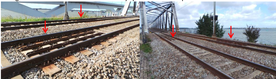
Figure 6.11. Expansion joints on the right side of the bridge.
