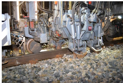
Figure 4.11. Tamping in a transition zone.
