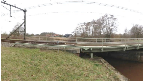
Figure 6.1. A typical track transition zone in the Netherlands.
