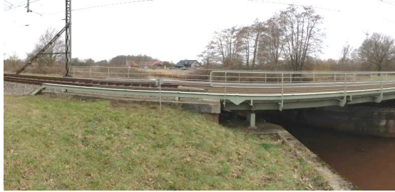
Figure 5.1. A typical bridge transition zone.
