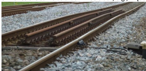
Figure 5.16. Transition zone with large track irregularities.
