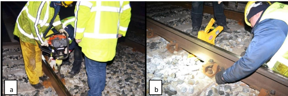
Figure 4.12. Adjustment of the fasteners.
