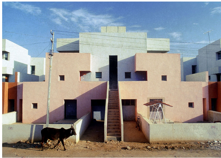
Life Insurance Corporation Housing – photo courtesy of VSF
