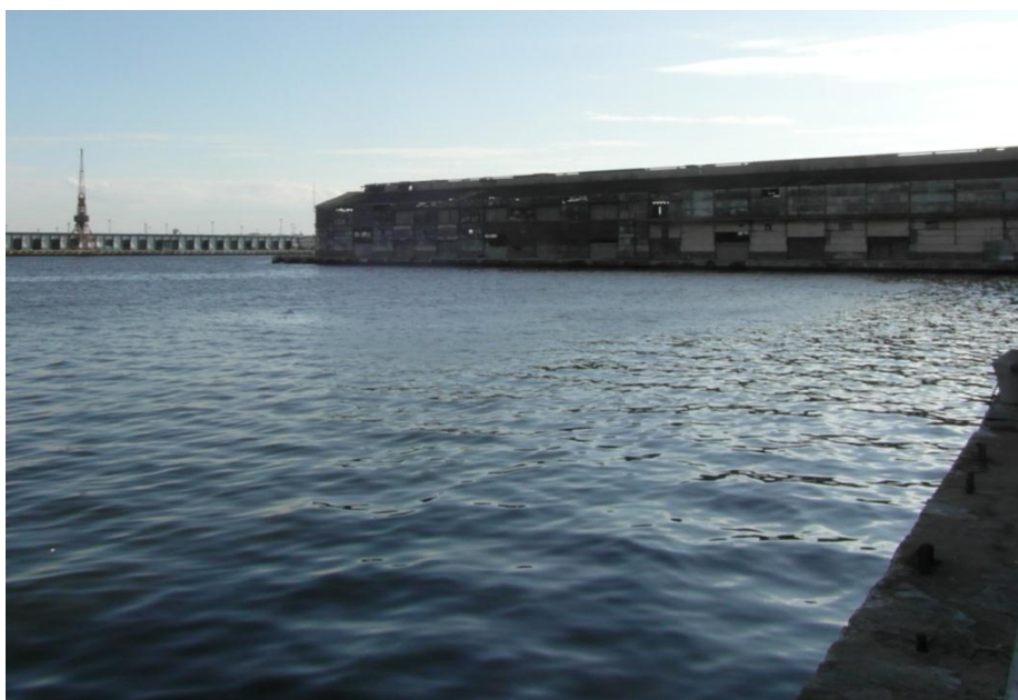
figure F.5 – the Espigón Aracelio Iglesias as seen from the Almacén San Jose (02/09/2013)
