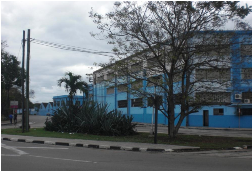
figure F.15 – the street side of the terminal Díaz no. 1 with left a part of the warehouse of Díaz no. 2 (03/02/2013)
