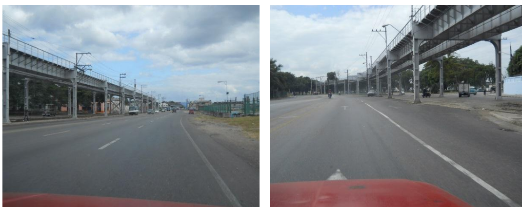
figure E.2 – Avenida del Puerto between Arroyo and the bus station. On the left eastwards to Habana Vieja. On the right westwards towards Castillo de Atarés, with the right turn onto Arroyo.
