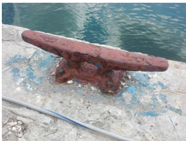
figure O.16 – an example of a cleat, Marina Hemingway (02/22/2013)
