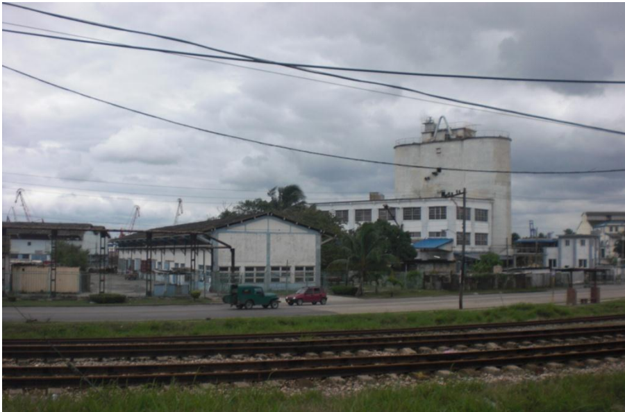
figure F.23 – several facilities at the Muelle Osvaldo Sanchez (03/02/2013)
