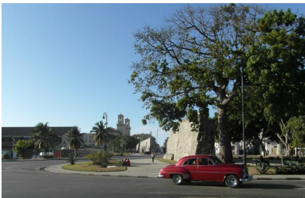
figure C.16 – old city wall
