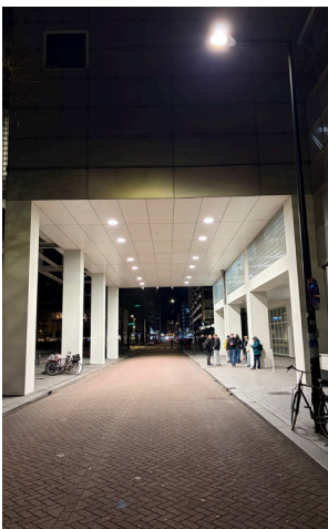
Figure 43. The theatre hangs over de street, creating a covert entrance.
