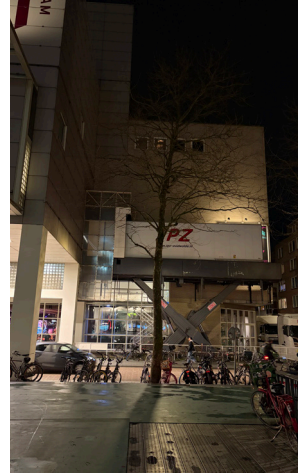
Figure 42. At the front façade there is a truck lift.
