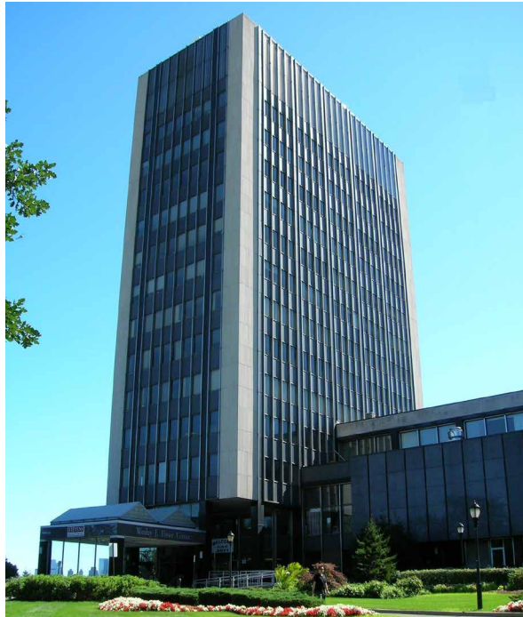
FIG. 6.1 The Wesley Howe Center at Stevens Institute of Technology is an example of first generation curtain walls buildings that need significant building systems upgrades.
