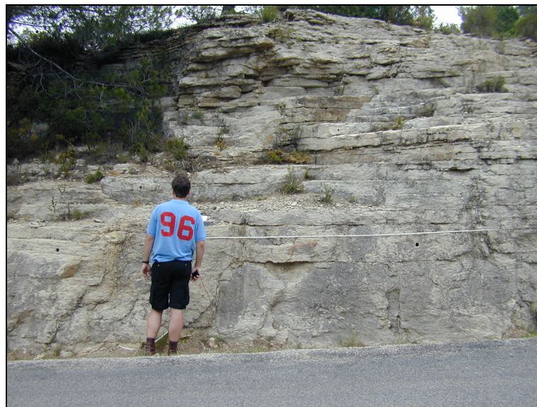
Figure 2.1. An example of integral bedding discontinuities that become mechanical discontinuities due to a combination of stress relief and weathering (solution). This is a man-made slope in Lower Muschelkalk (Triassic) Limestones, beside road T322, near the town of Colldejou (Photo: W. Verwaal, 2001).
