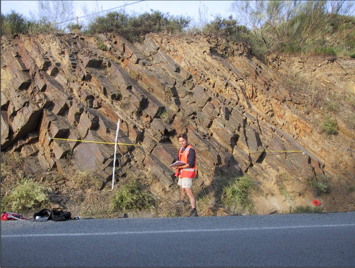
Figure 11.3. Position of the horizontal (yellow tape) and vertical scanline (white ruler) at exposure of Bellmont site. The horizontal scanline survey was done from left to right over 6.45 metres.
