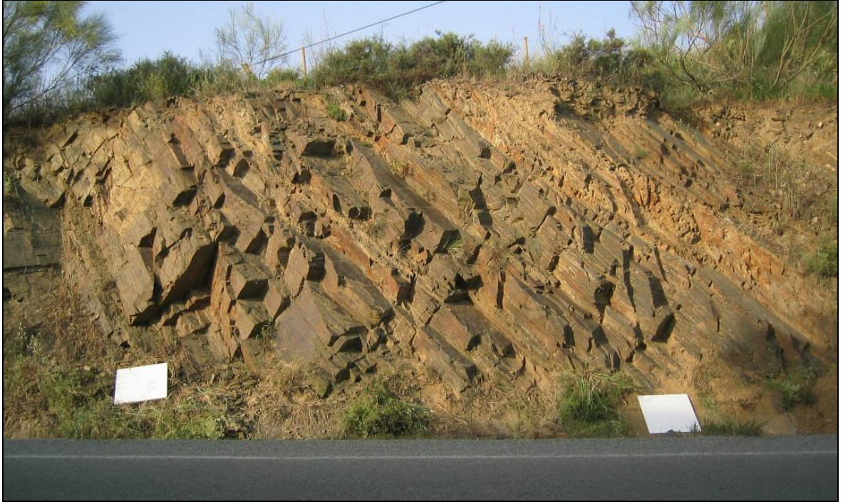
Figure 5.4. Photograph of the surveyed and scanned rock exposure at Site 1. The two white boards act as scale and orientation reference: the left white board has an orientation of 024/40 and the right one 022/39. Both white boards are 60 x 60 cm in dimension. View direction is SSW.
