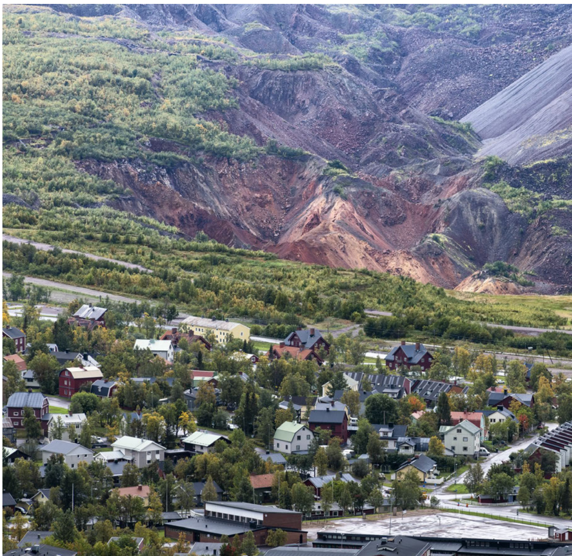
Ground caving due to underground mining in Kiruna [Photograph by Lennart Durehed - Arkdes, 2019]
