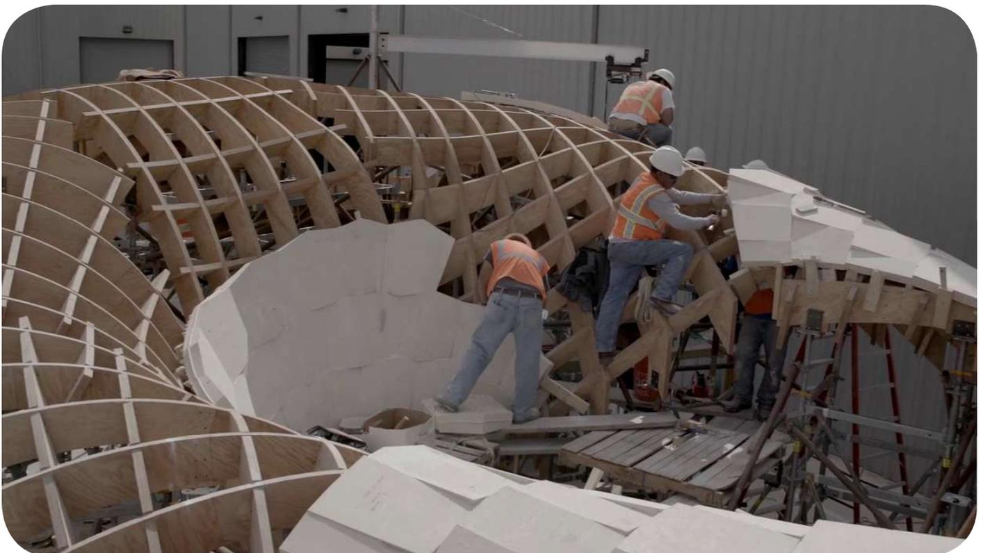
Figure 157. Wooden support structure used for construction of the Armadillo Vault (Arthur, 2017)
