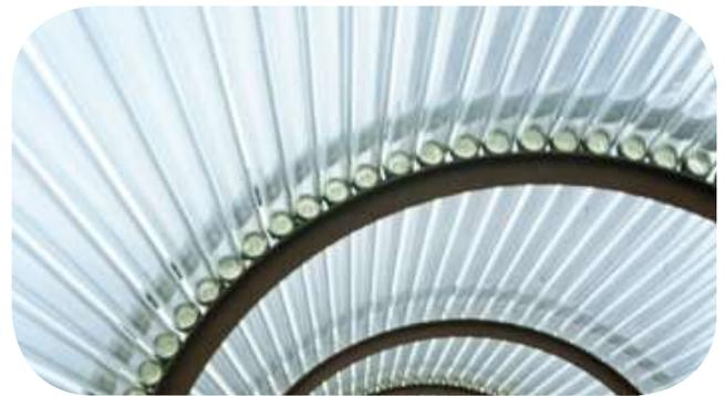
Figure 106. Extruded glass used as a vault (Borum, n.d.)
