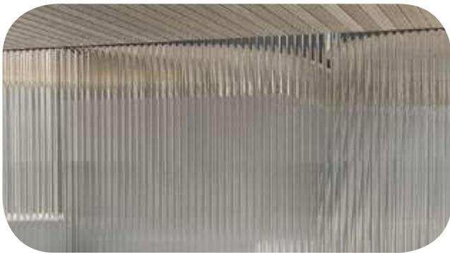
Figure 105. Extruded glass used as a wall application (source: www.evstudio.com)
