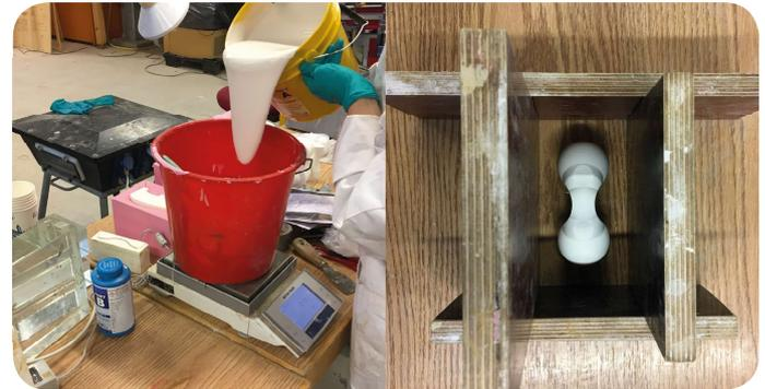
Figure 164. (left) weigh the part A and B, (right) wooden box and clay fixation
