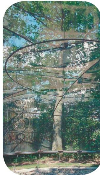
The glass dome at ILEK is an example of chemically strengthened glass.
