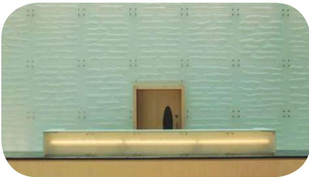
Example of textured float glass where an additional layer is added by heating the float glass and melting a fire resistant substrate.
