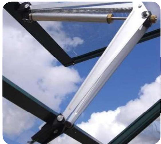
Figure160. Window clamps that react to temperature differences (source: www.tuinkassenwinkel.nl)
