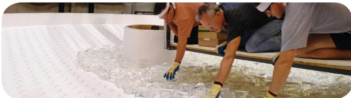
Figure 84. Preparation before casting: the honey comb mold (source:www.gmto.orgs.co.uk).
