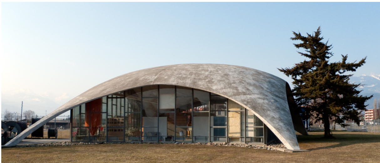
Figure 1.4 Heinz Isler, 1968: Laboratory and research facility for the Gips Union; panoramio.com
