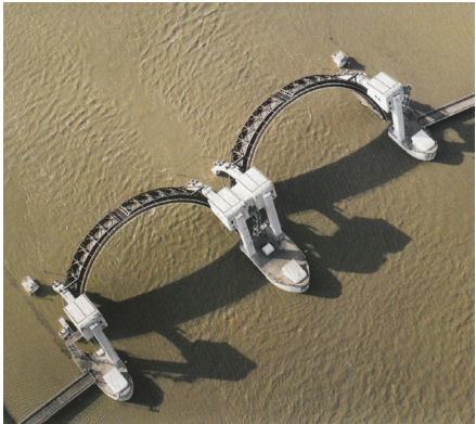
4.1.9 The weir at Driel in the river Nederrijn-Lek. Some weirs have more impact on the flood risk system than others: the Driel weir can be raised to improve navigation or to lower resistance for high water discharge. Regular weirs like in the river Meuse and upstream in the in the Rhine cannot do this (they can be opened for high water discharge, but ships always have to pass through locks).
