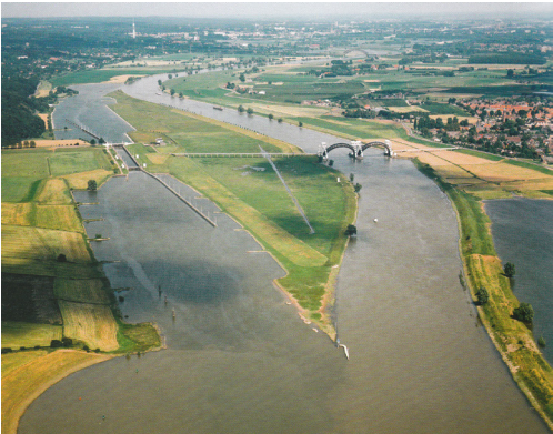
4.1.9 The weir at Driel in the river Nederrijn-Lek. Some weirs have more impact on the flood risk system than others: the Driel weir can be raised to improve navigation or to lower resistance for high water discharge. Regular weirs like in the river Meuse and upstream in the in the Rhine cannot do this (they can be opened for high water discharge, but ships always have to pass through locks).
