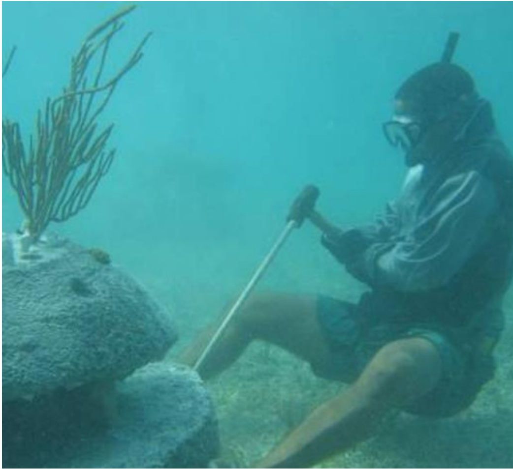
Figure L6: Foundation pile installation on a layer cake element
