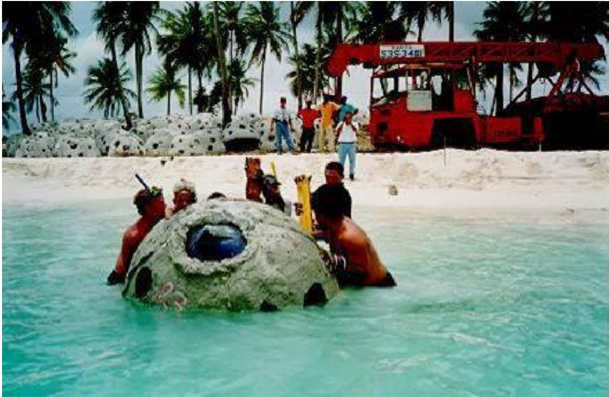
Figure L3: Floatation of the Reef Ball TM
