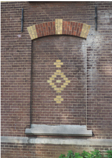
Fig.: Blind window frame 'Grote Boerderij'
