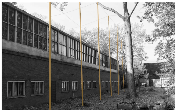
Fig.: 11 lightning catchers spanning the former ammunition factory
