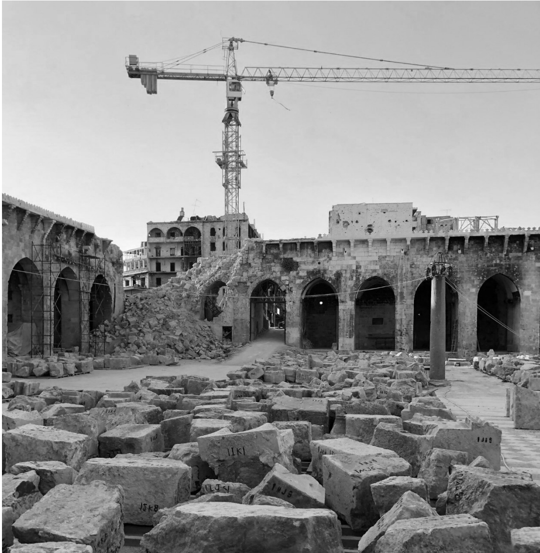
Figure 28. Damage to the Great Umayyad Mosque of Aleppo, including damage to the minaret., by Francesco Bandarin, 2013
