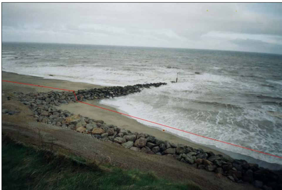
Figure 18 Permeable Rock groyne at Mappleton
