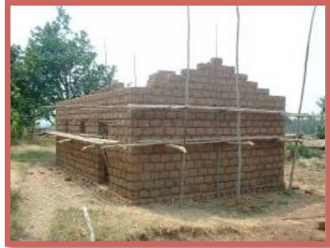
Figure 10 Timber framed house filled with clay (personally taken photo) Figure 11 Adobe house (personally taken photo)
