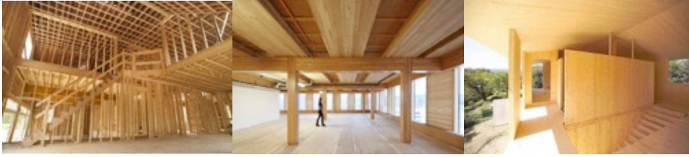
Figure 67 Timber structural systems - platform, framed and panelized
