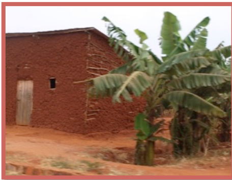
Figure 10 Timber framed house filled with clay (personally taken photo) Figure 11 Adobe house (personally taken photo)
