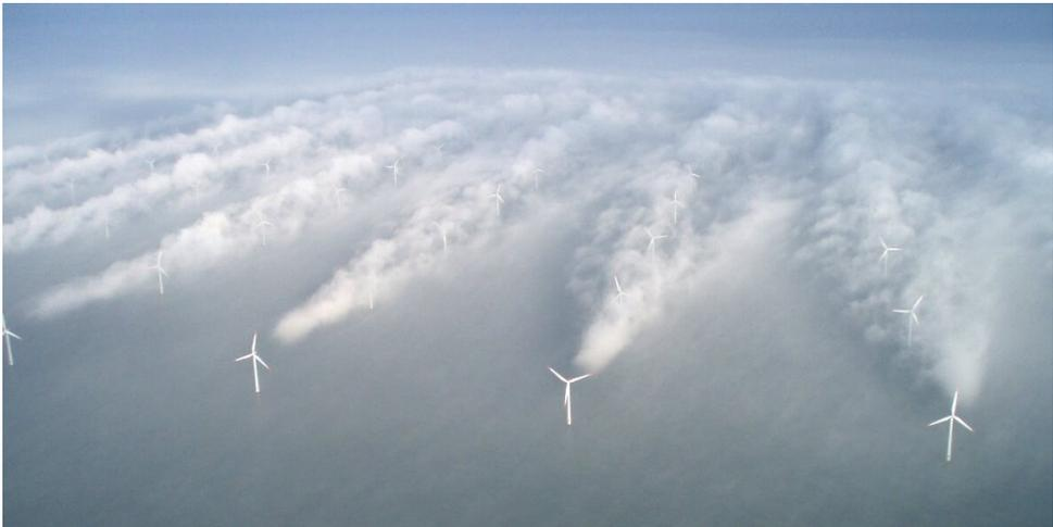
Figure 1.6: A famous photograph by Christian Steiness of the Horns Rev wind farm in Denmark, which clearly shows the wakes behind turbines. The downstream rows of turbines experience lower wind speeds and higher turbulence intensities as a result of the operation of the upstream turbines.
