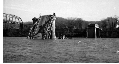
Figure 1.1: Impacts of corrosion. (a) Aloha airlines disintegration. (b) Silver Bridge collapse [1, 2]
