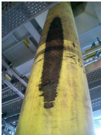
Figure 1.5: Damaged outer sheath (Crome, 2013)
