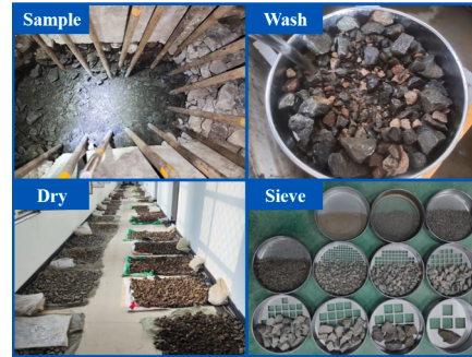
(b) determine the kinds of ballast bed defects through on-site excavation.
