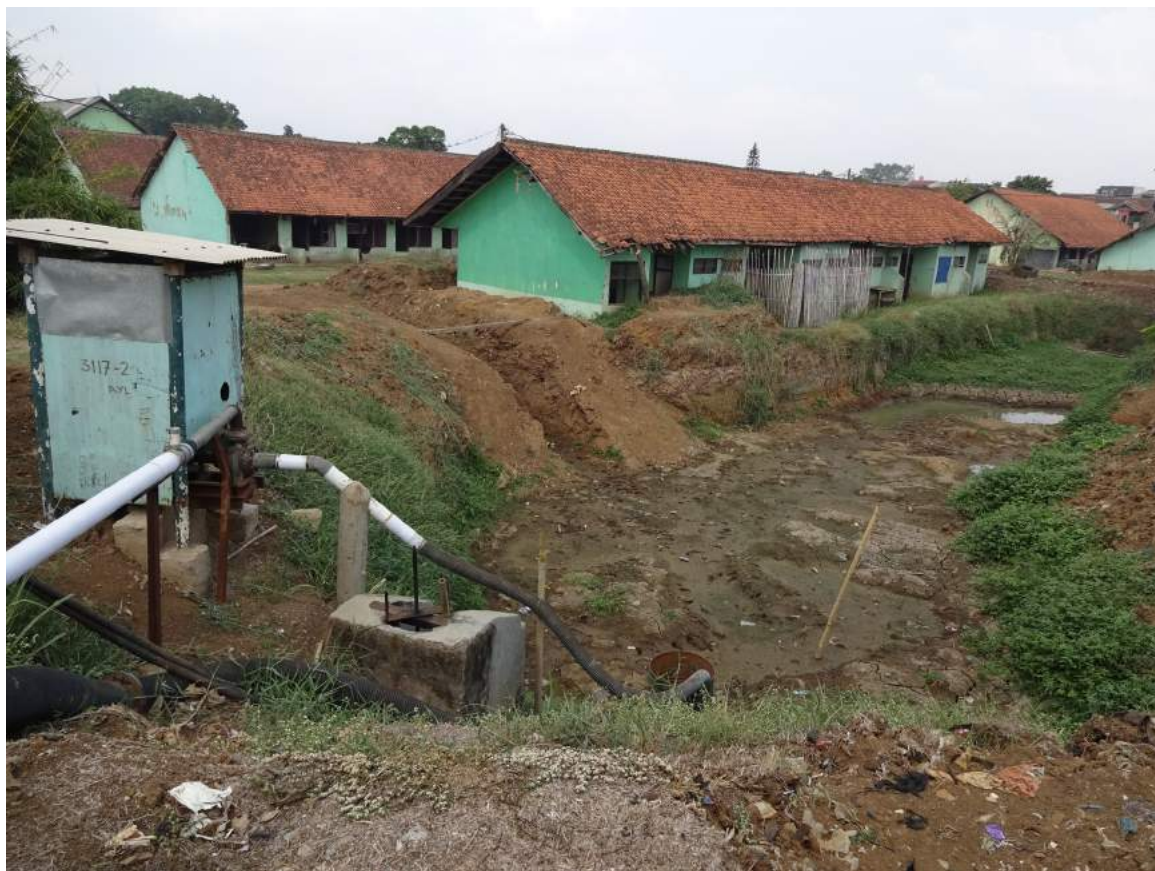
Figure 49 Overflow and pump station in the military area Source: Author
