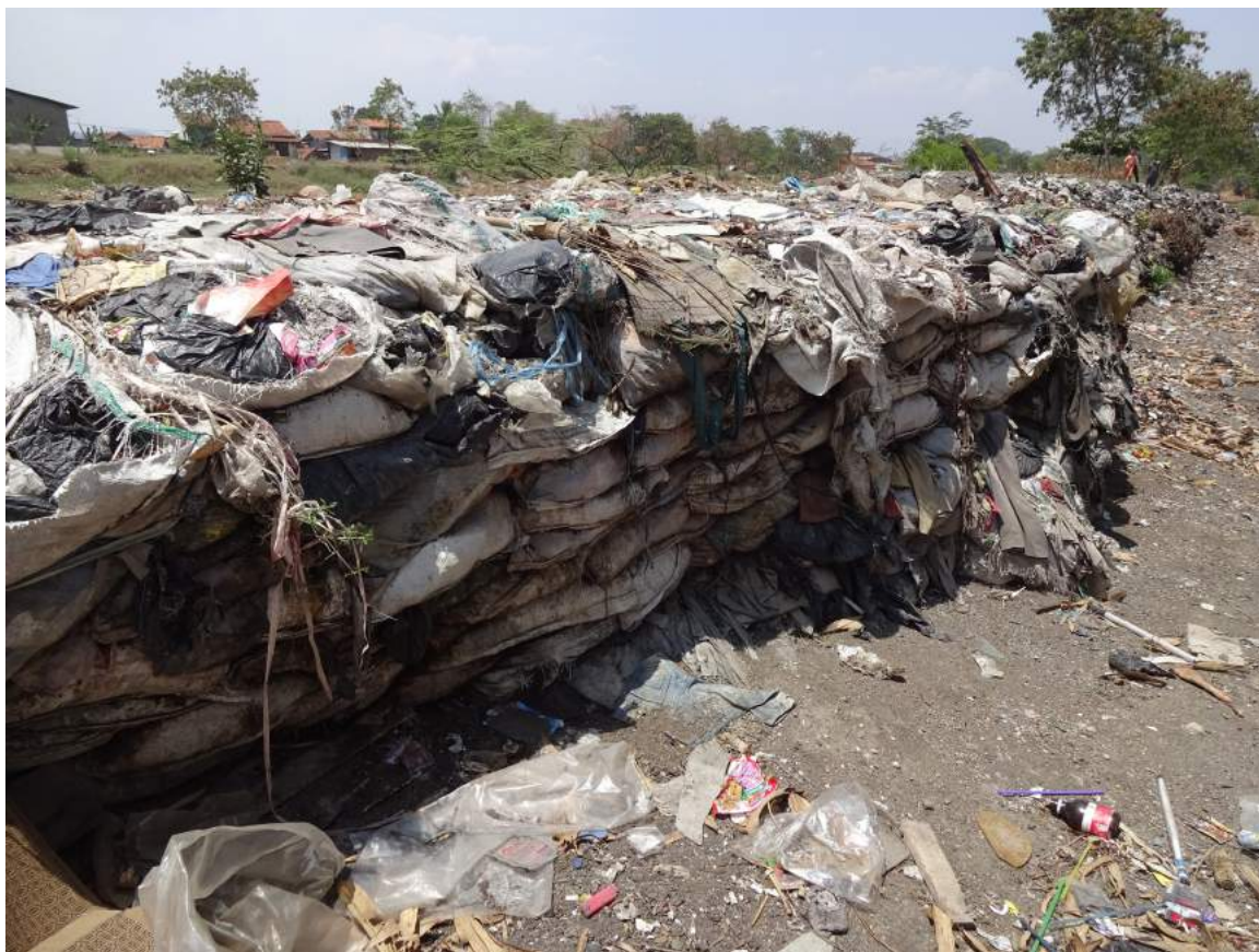
Figure 40 Repairs of the existing dike failure due to landslides Source: Author
