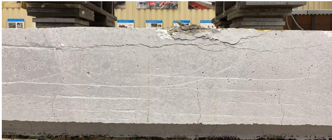
Fig.3.33. LB3. Mid-span from south side after testing showing cracks and crushing.
