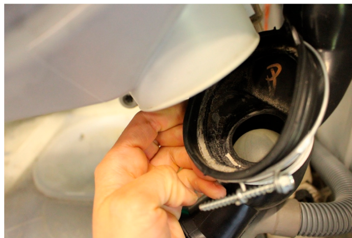
Figure 4. Shallow connection with minimum overlap (approx. 5 mm) between the tub outlet and its corresponding hose. Shallow connections can be vulnerable or cause reassembly issues despite the reusable connector, potentially leading to leaks. In this case, a leak from the tub outlet hose could cause a short circuit since it is positioned directly on top of the pump.
