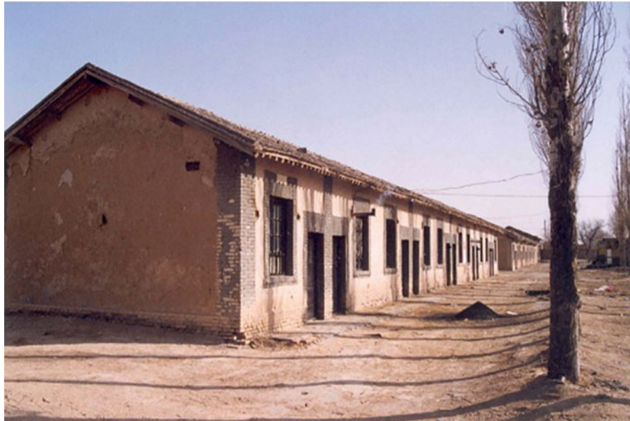
FIG. 9.1 A Variation of Scientific Gandalei Using Brick Columns and Brick Door Frames. Source: Penglin Zhu (Collected during the fieldwork).
