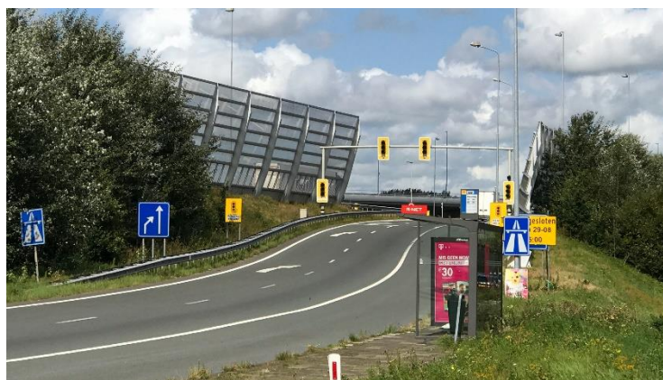
Figure 2-12. Photo ramp metering at A10 Basisweg (location A10Re 27.3b)
