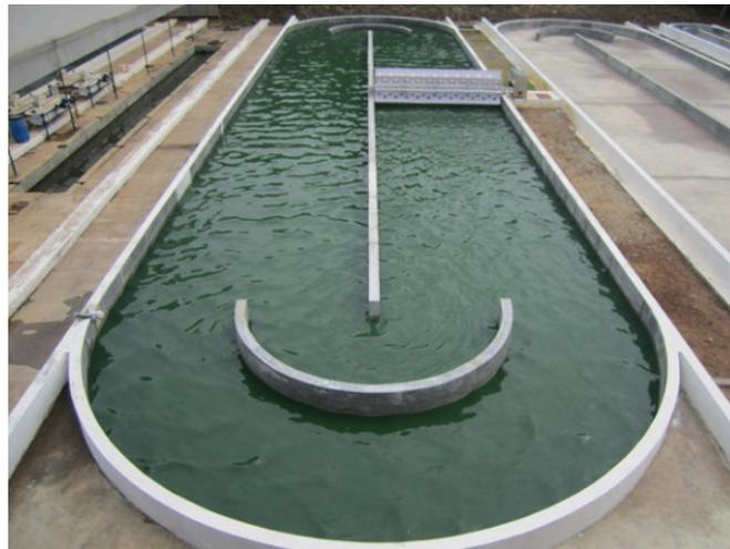
**Figure 4-3:** Typical example of a raceway pond
