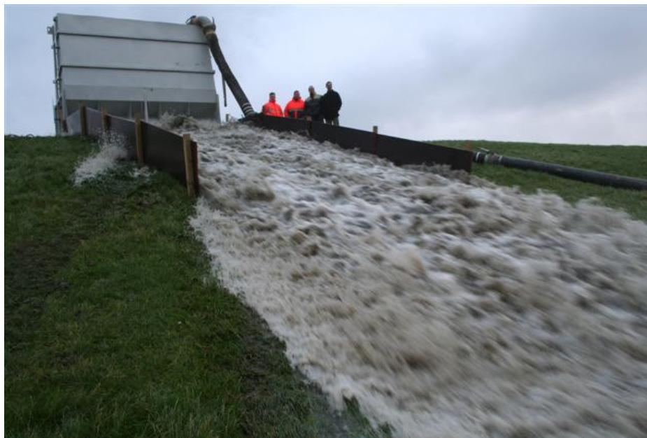
Picture 7.15. The first water flowed over the dike on 20 December 2006.
