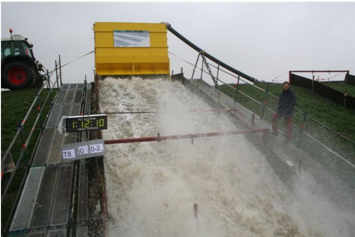
Picture 8.7. Release of a large volume during test with 50 l/s per m. Hose of pump was put directly into the box of the simulator.
