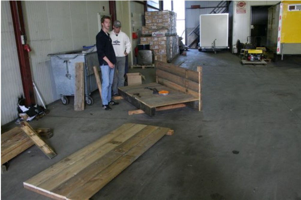
Picture 4.3. Construction of 2 m long and 1 m wide calibration flume
