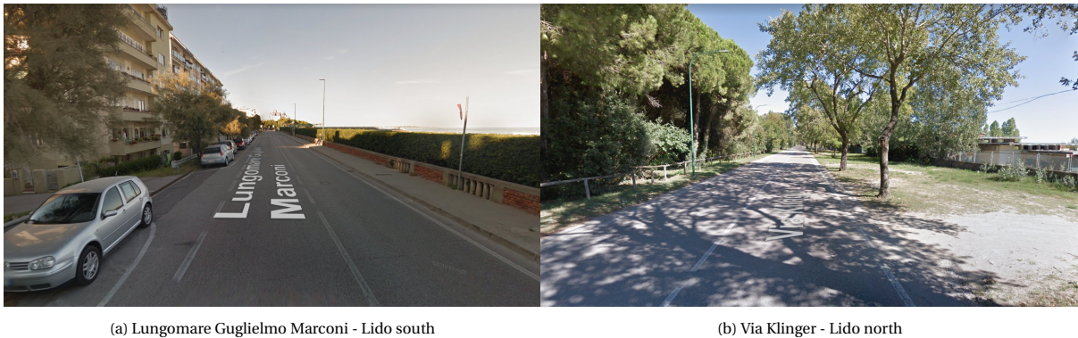
Figure D.2: Two pictures showing the different landscapes of the Lido flood defence system [21].
