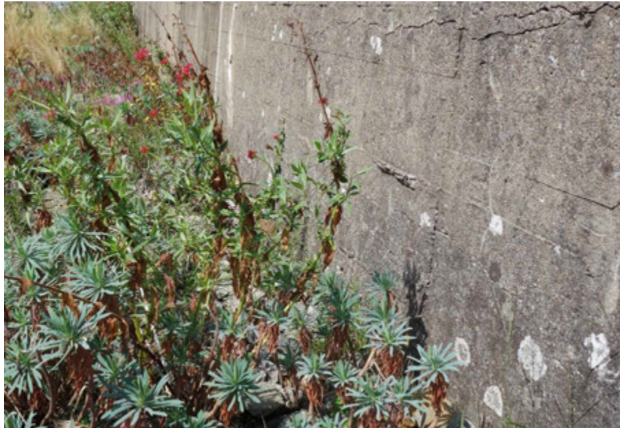
FIG. 5.25 The plants and the concrete wall
