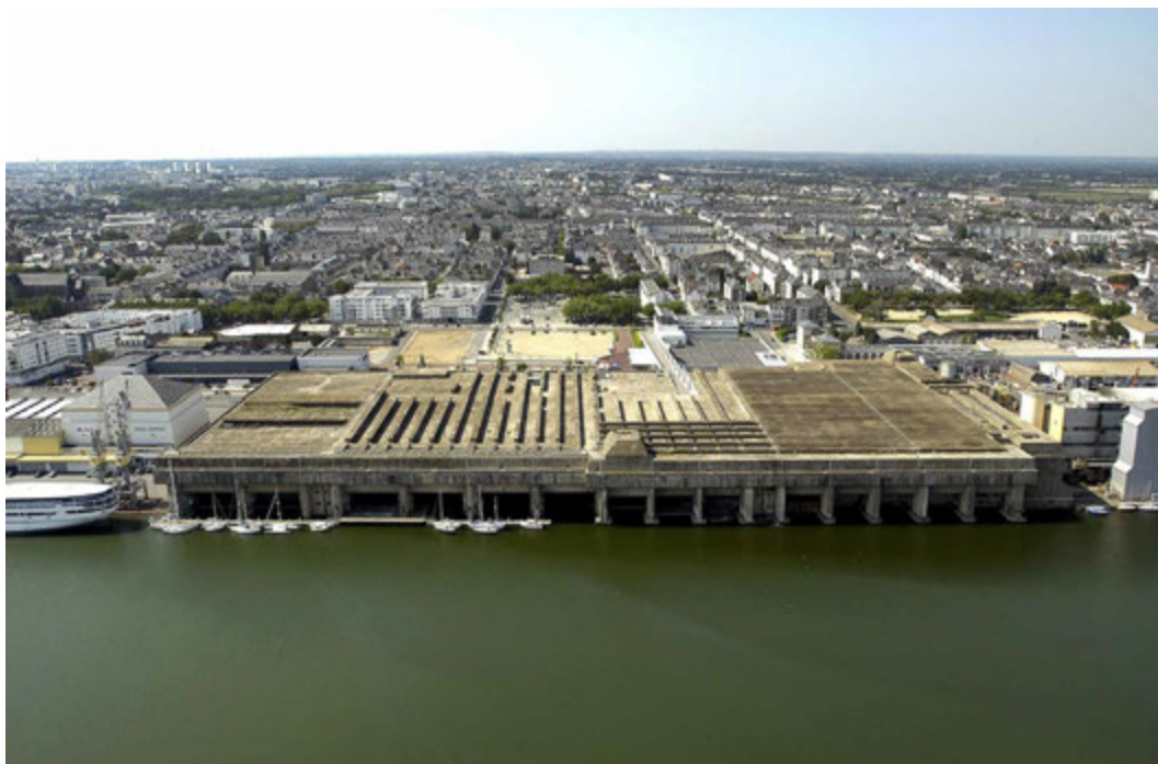
FIG. 5.7 The aerial image of the roof
