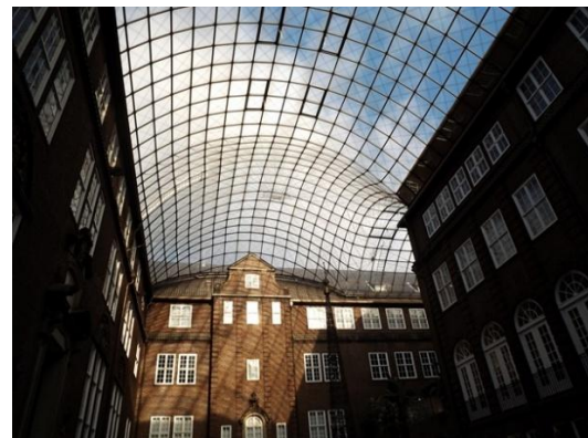
Figure 17: Courtyard Roof of the Museum of Hamburg (Source: Ermias Y., 2013)
