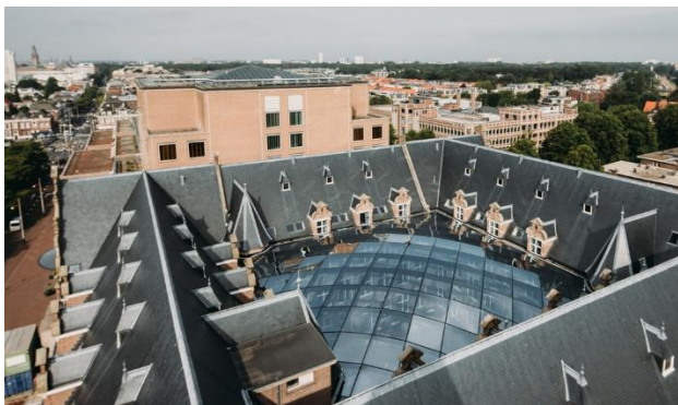
Figure 82: Overview of the C30 structure. (Source: Octatube, 2020)
