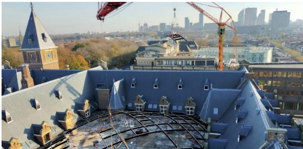
Figure 85: Placing of the ladder frames using cranes. (Source: Octatube, 2020)
