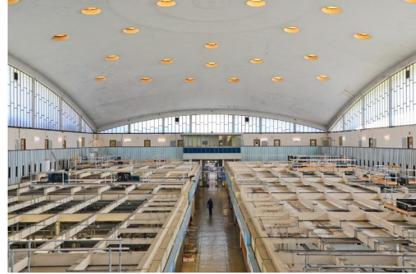
Figure 5: Ove Arup - Concrete shell roof for the Smithfield Poultry Market, London, UK. (Source: Julian Harrap Architects).
