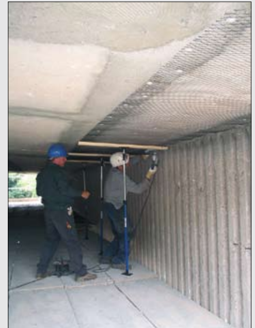
An already affected object has to be protected cathodically, that's why it's put in a web of titanium which later on is covered by a protective layer. The 'web' then just will function as an anode.
