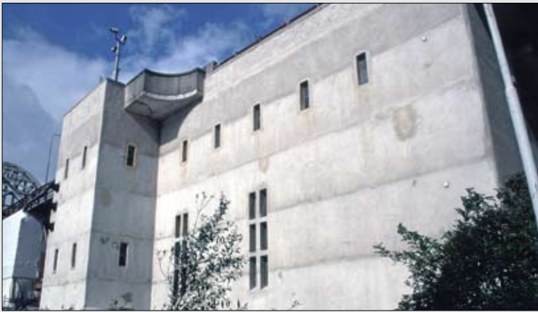
The bascule building of the Noord Bridge was fitted with cathodic protection in 1996, when the concrete was found to be severely affected. Even so, very few structures in the Netherlands use this type of protective technique.
