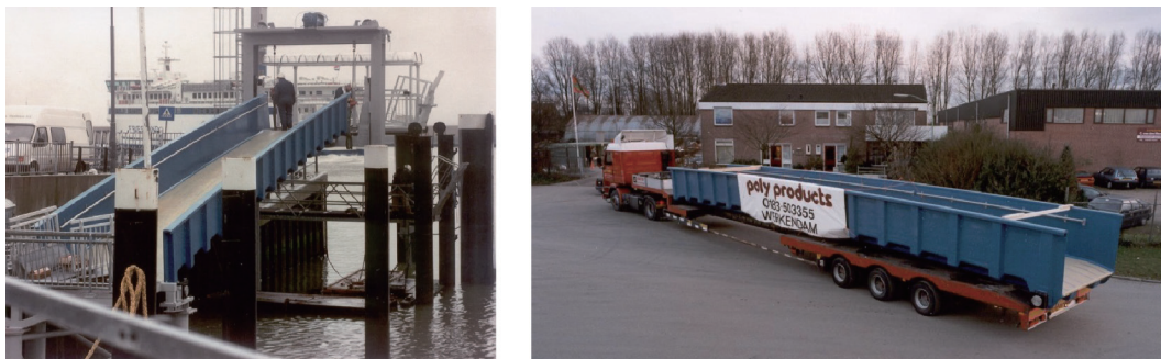
Fig. 3. Footbridge in Harlingen, the Netherlands (Poly Products, 1997).
