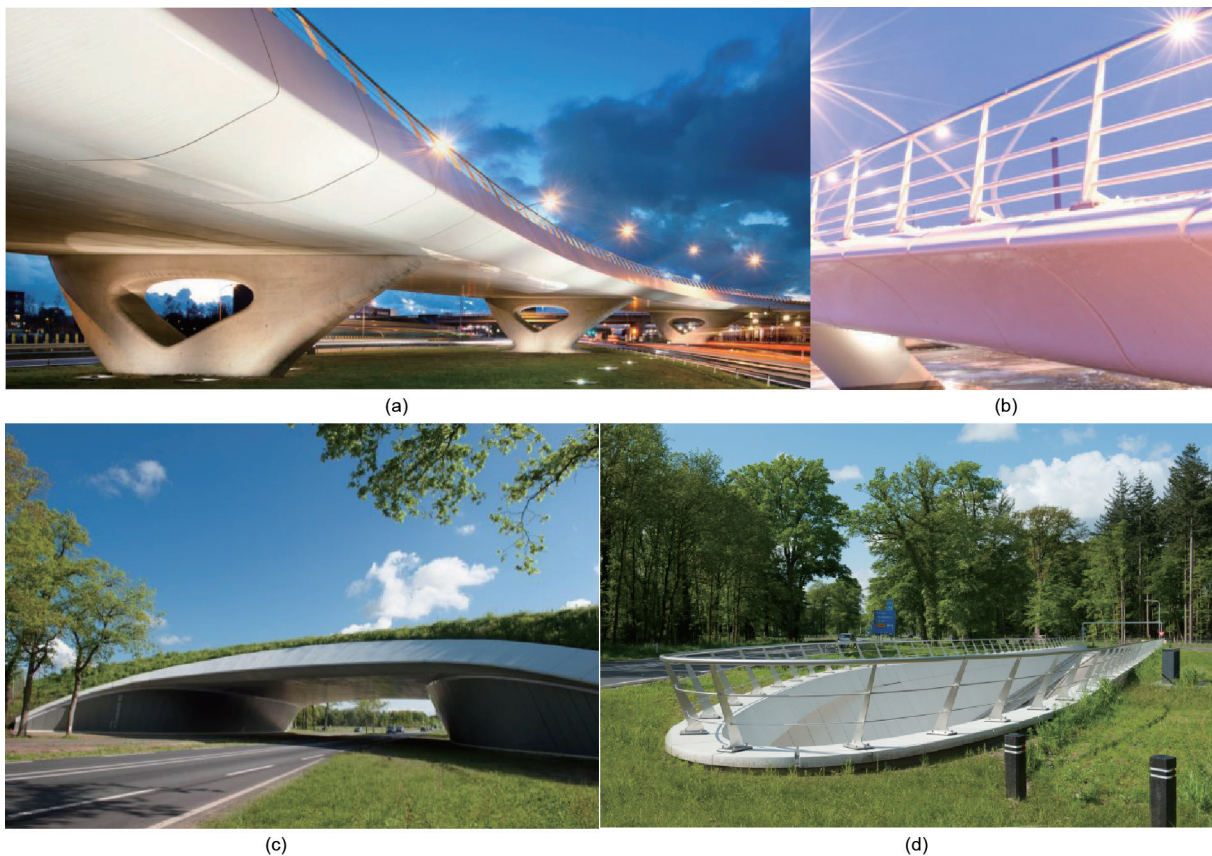
Fig. 9. Some projects in the Netherlands with FRP edge elements. (a) The fly-over Waarderpolder in Haarlem; (b) edge elements on the Juliana Bridge in Zaanstad; (c, d) the wildlife crossing and tunnel in Rijssen-Wierden (Royal HaskoningDHV, 2007, 2013, 2013).
