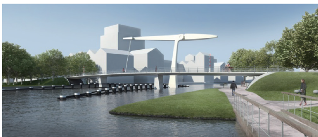
Fig. 13. A design for a monocoque FRP drawbridge for pedestrians and bicycles across the Rhine in Katwijk (Royal HaskoningDHV, 2014). (a) Cross section of the deck (unit: mm); (b) artist impression.
