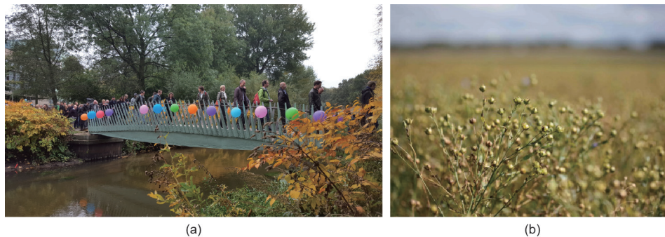
Fig. 21. Flax fibers, bio-resin, polylactic acid (PLA) foam, and natural cork were used to produce the bio-composite bridge in Eindhoven. (a) The opening of the bio-composite footbridge in Eindhoven (copyright by the author, Oct 27, 2016); (b) the flax plant from which stems the flax fibers are extracted.
