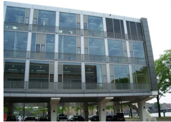
MARINE 70'S BUILDING Recently renovated Government/navy office building
