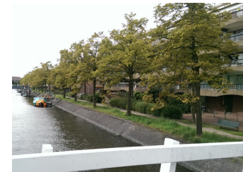
KATTENBURG DWELLINGS Social housing Dwellings at waterfront have the highest quality and fits into the loop masterplan, but they still need drastic transformation
