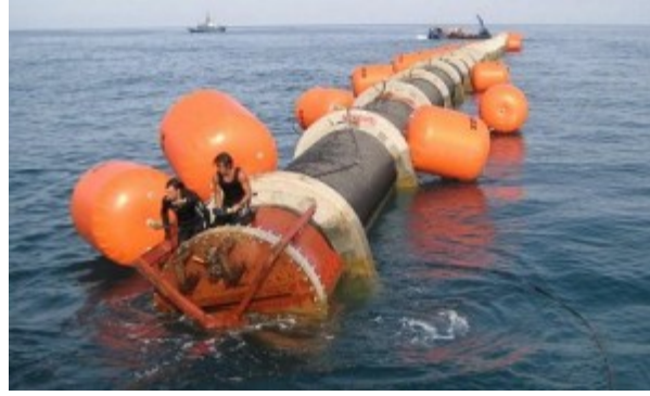
Figure 4.1: HDPE pipe installation with added shallow water buoyancy bags [41]
