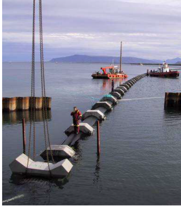
Figure 3.3: HDPE pipe with concrete weights before installation [30]
