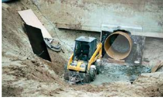
Figure 7.3: The discharge pipe of STP Houtrust [34].
