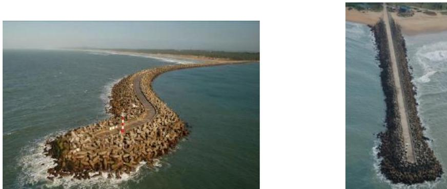
Figure 1.2 – South and North breakwaters and North of Richards Bay Port
