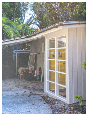
Figure 40. Photo of the entrance of Sharp House.
