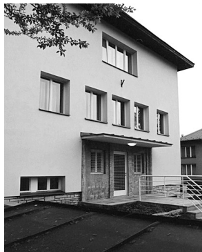
Figure 39. North facade and entrance of Villa Holzner.
