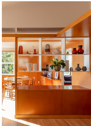
Figure 34. Photo of the cabinet connects to the ceiling.
