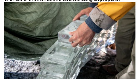
8. Placement of brick using manual pressure
