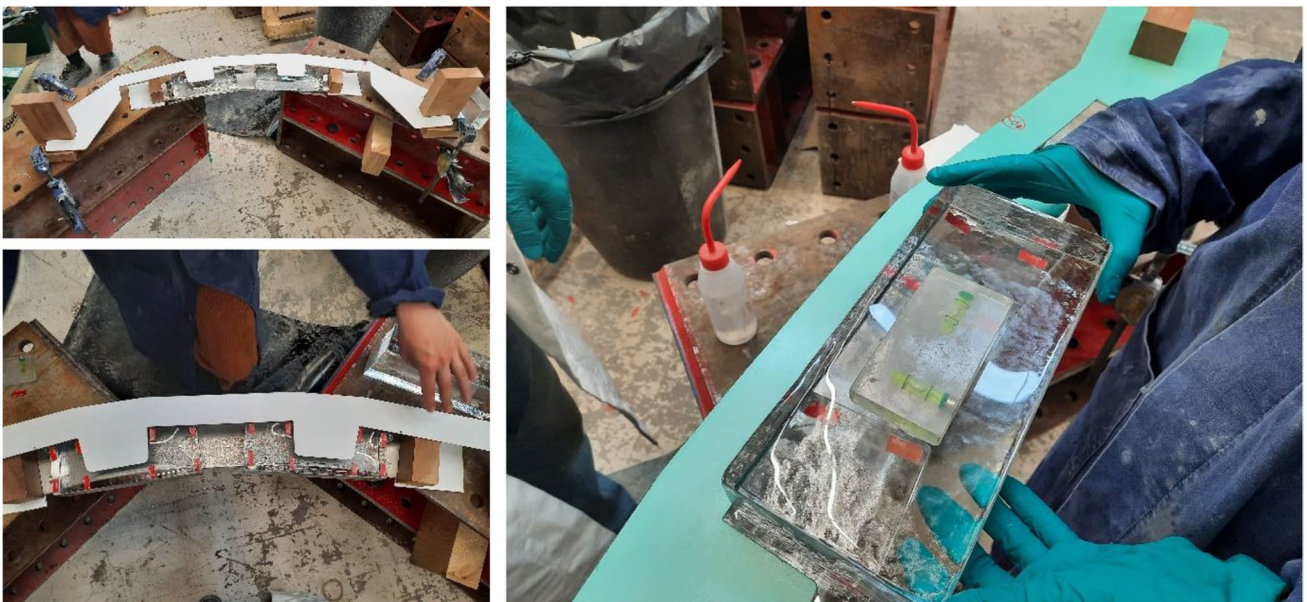
Fig. 16 Templates and wooden guides used to indicate the correct position of the glass bricks (left). Levelling of the glass brick with the help of a water-level and additional 0.5 mm double-sided tape stickers (right)
