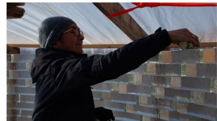
2. Bricks of the bottom layer are cleaned
