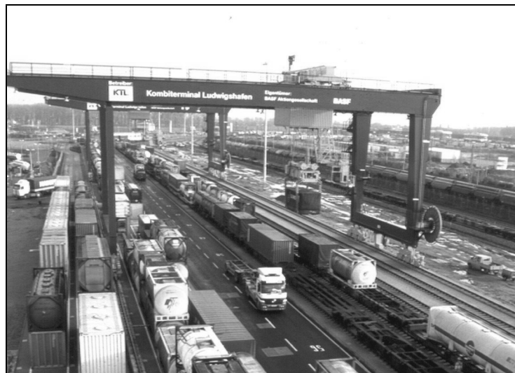
Figure 3–8: An example of a road-rail terminal: KombiVerkehr terminal in Ludwigshafen
