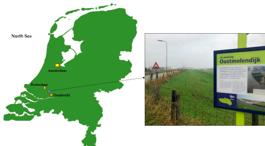
Figure 7. Location of the case study embankment Oostmolendijk.
