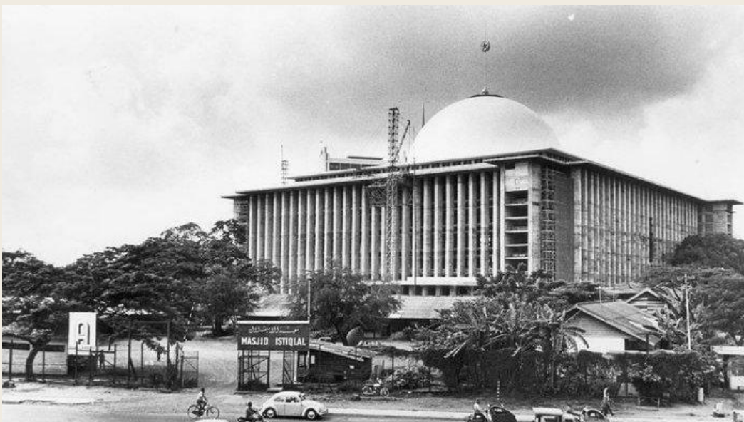
Figure 4: Istiqlal Mosque during construction, c. 1950s. Image retrieved from istiqlal.or.id
