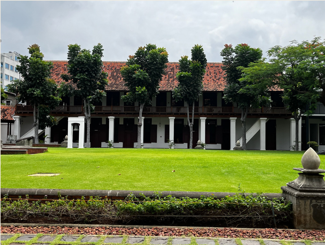
Figure 16: Courtyard of Gedung Arsip Nasional , 2025. Own photo Image taken during personal site visit
