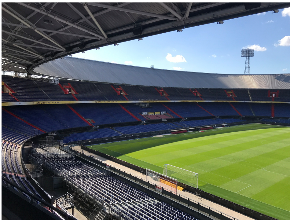
Figure 1.2: The two oval tiers of the grandstand in the Feyenoord Stadium, the lower demountable section and the roof of the stadium, from (Feyenoord, 2017b)
