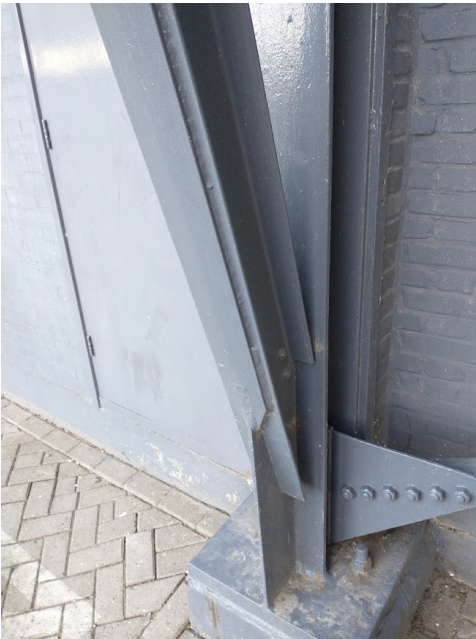
(a) The connection of the spine to the base
