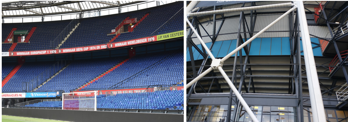
(a) Front of both rings, from (Voetbal Rotterdam, 2020). The transparent wall on the left is placed above a dilatation joint. (b) Back of the first ring and trusses (own work)
