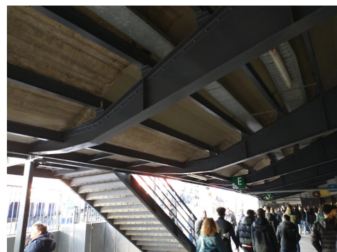
(f) The beam supporting the lower cantilever
