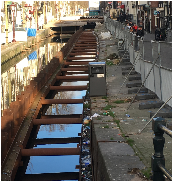
Figure A.1: Quay wall on the Oudezijdse Achterburgwal showing large horizontal displacements, photo taken by author on 3-1-2019
