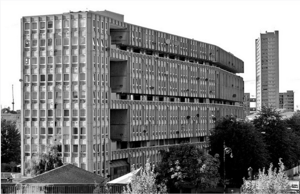
Figure 13. Robin Hood Gardens Estate in Poplar, Tower Hamlets. Image credit: https://londonist.com/2012/03/robin-hood-gardens-set-for-demolition
