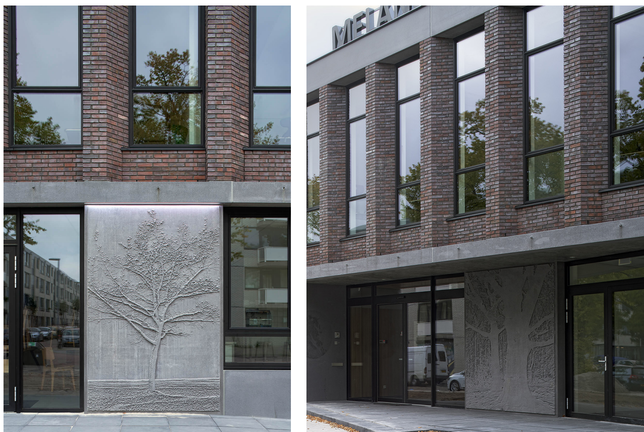
Fig 9.8: Deep set windows with side-fins and overhang as design strategy. Source: KAW Architects
