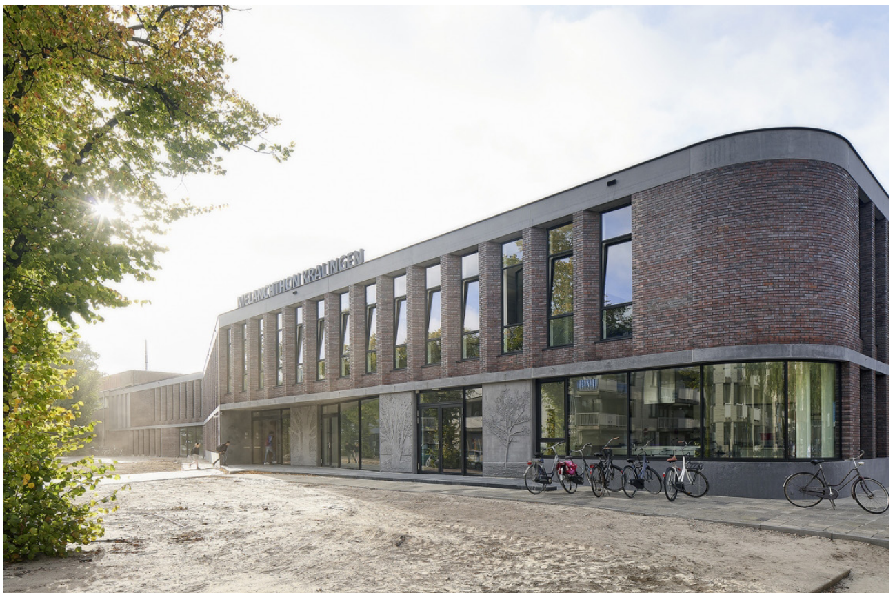
Fig 9.6: Melanchthon School, Rotterdam. Source: KAW architects.
