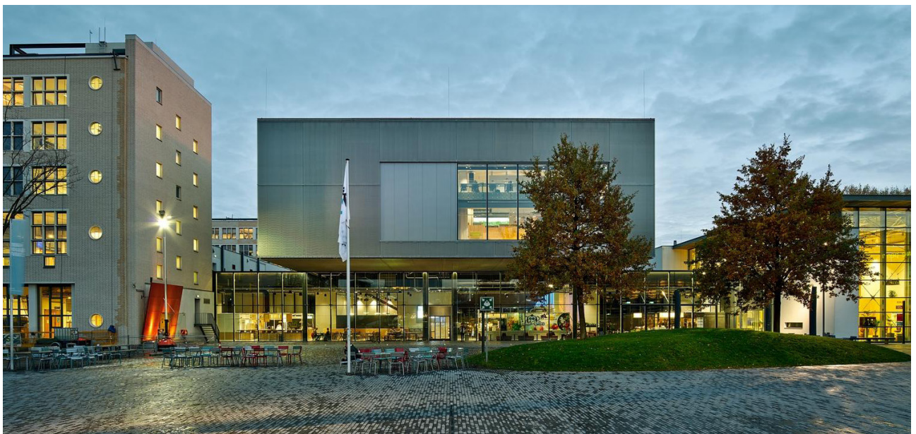
Fig 9.1: Pulse Building, TU Delft Campus . Source: qbiqwallsystems.com
