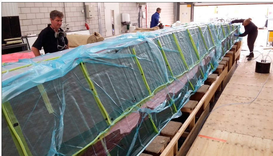
Fig. 4: Production of the 14m long bridge
