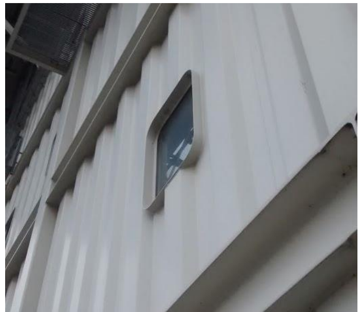
Figure 8: Offshore Accommodation External Wall (source; author)
