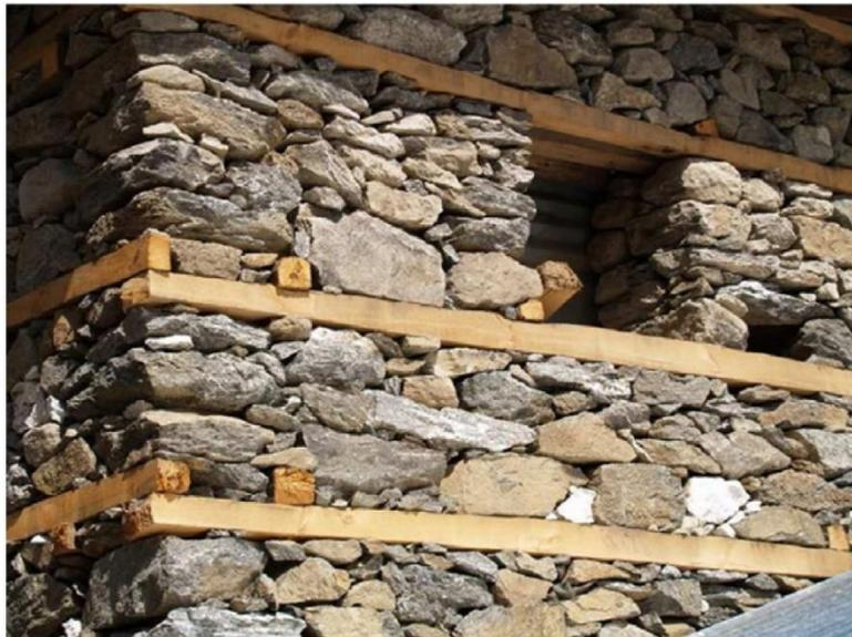
Appendix F : Wooden beams and dry stone masonry (Carabbio et al., 2018).
