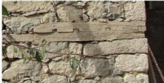
Appendix J : Vernacular joints found in Italy and Turkey using wooden pegs and flexible joints (Ortega et al., 2014 p. 7).
