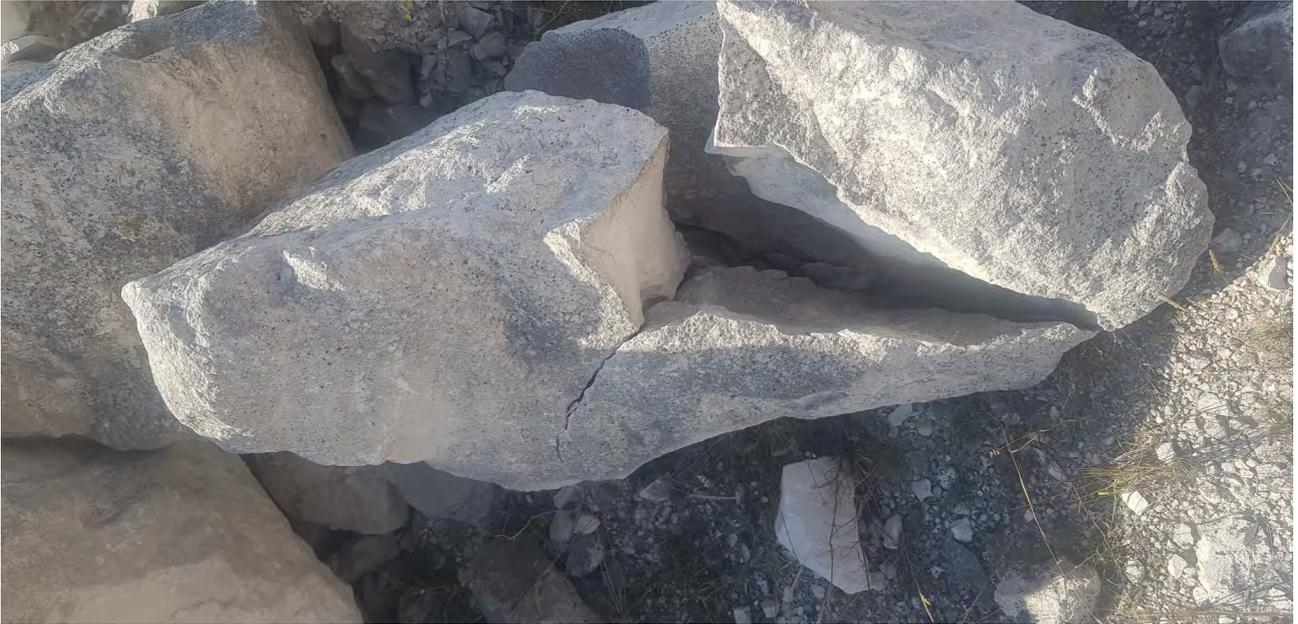
Figure E.17: Examples of damages of the large rocks in the pile
