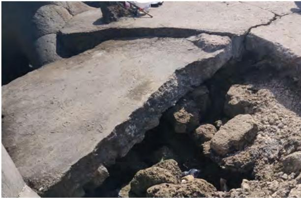
(a) Pieces broke off at the head of the concrete plates
