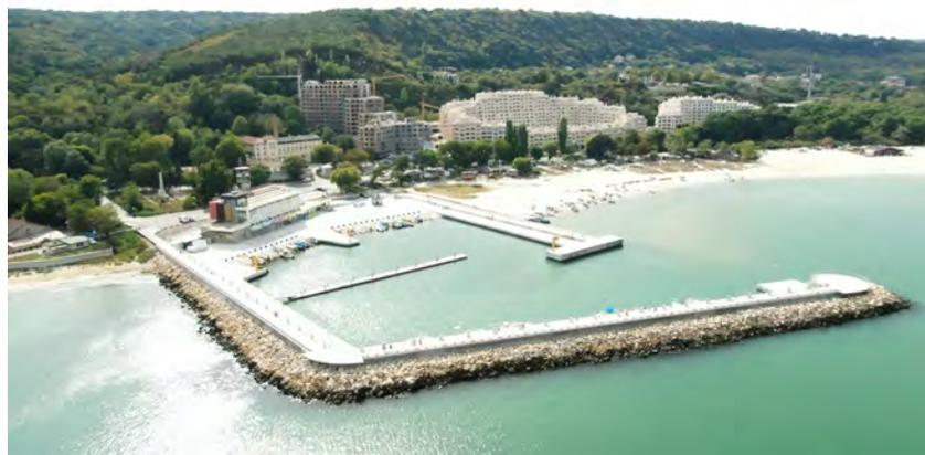
Figure 2.14: Breakwater at Karantinata Port
