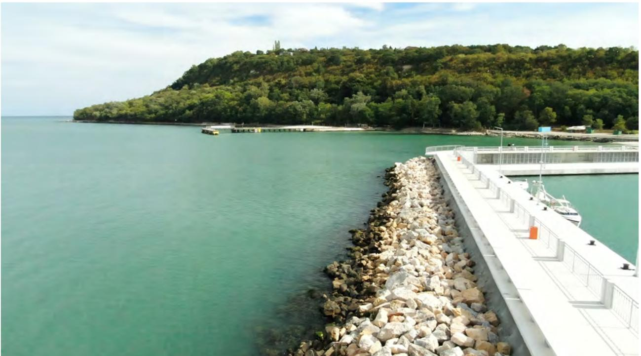
Figure 2.16: Seaside of the breakwater with plateau and steep slope
