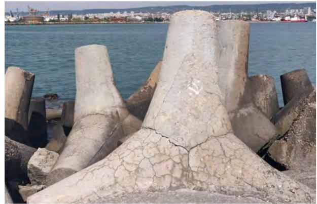
(b) Cracks in Tetrapods at head of breakwater
