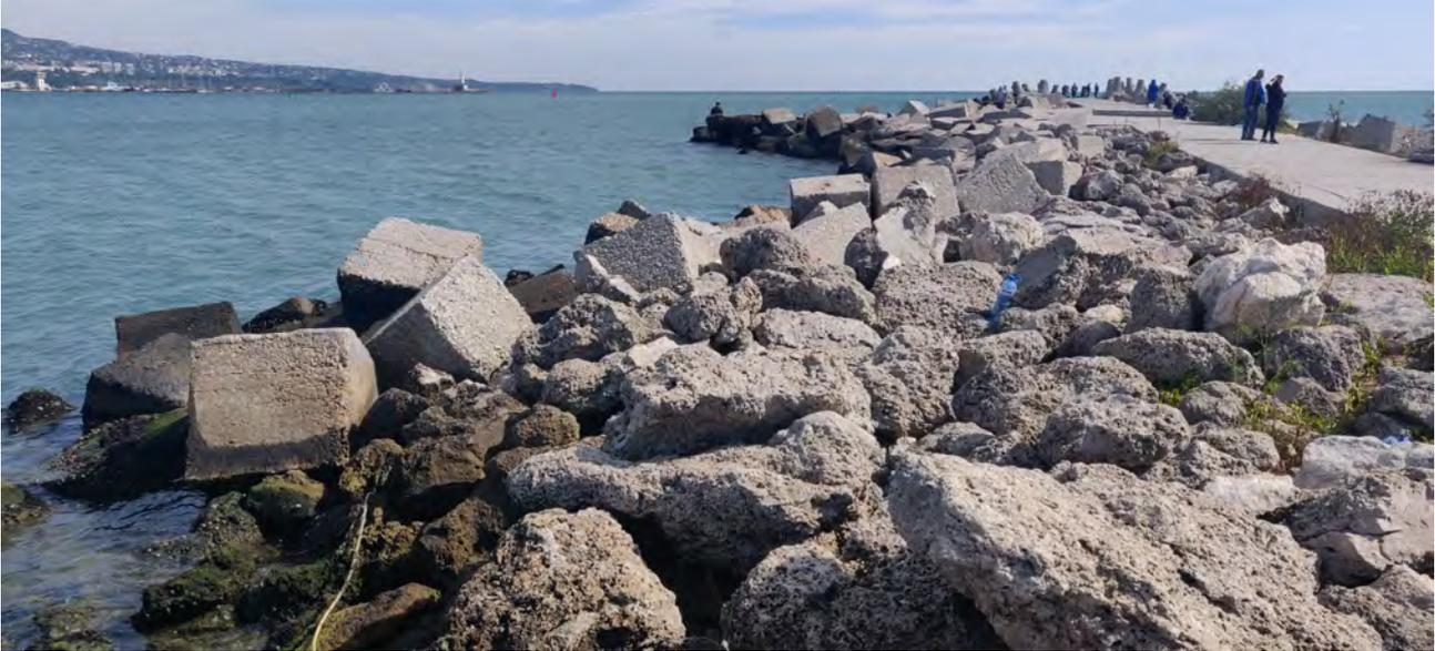
Figure 2.19: Rock and blocks sticking out at two places in the middle part of the breakwater
