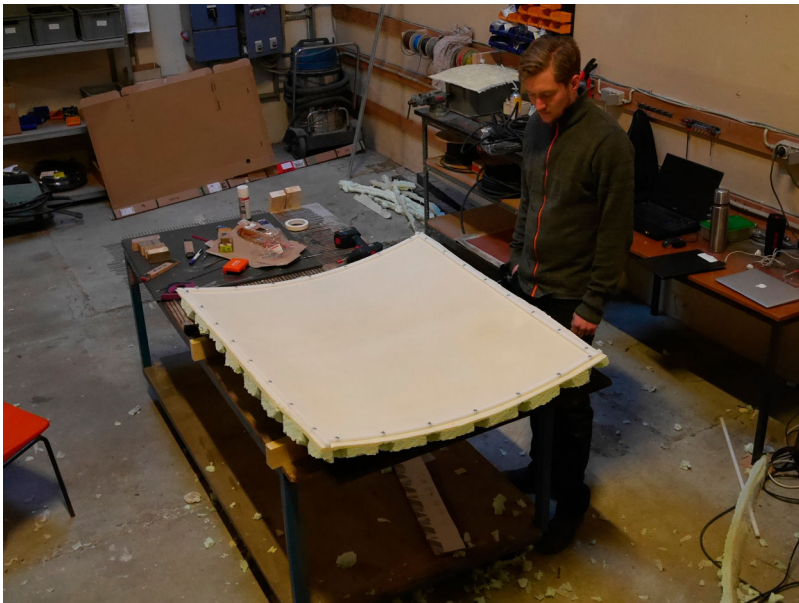
Figure 29. Finished intermediate mould ready for being tested with sprayed GFRc.
