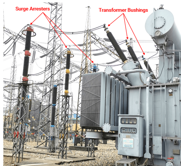
Figure 2.4: A power transformer accompanied by a surge arrester. [15]
